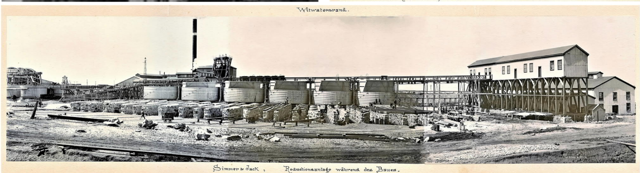
Photo 3: S&J mine during construction of production facilities 7
