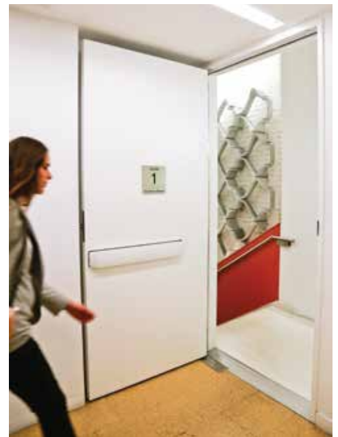
ABOVE: At the Bullitt Center in Seattle, Washington, natural materials and light make taking the stairs more appealing. (©Nic Lehoux) RIGHT: Electromagnets hold open doors to fire stairways at the Center for Architecture in New York City. (Emily Young)
