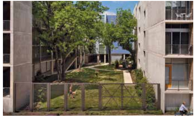
The 1221 Broadway project in San Antonio, Texas, offers a high-quality, fenced-in dog park as an amenity for residents. (Chris Cooper)
